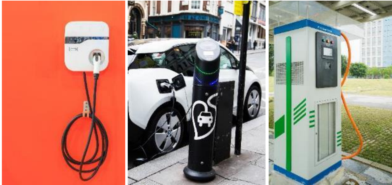
Figure 4: A domestic wall mounted charging point, a floor mounted charging point and rapid charging point 16
